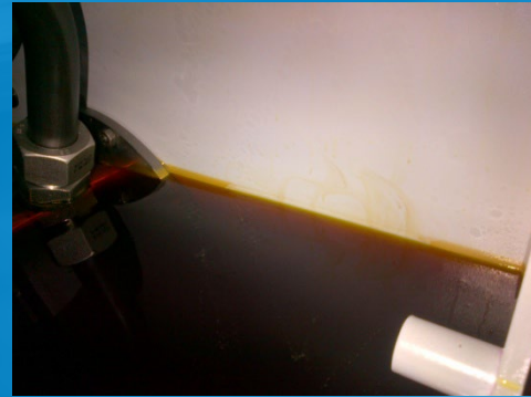
Varnish on the tank wall
